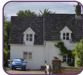
Pitched roof with dormers
