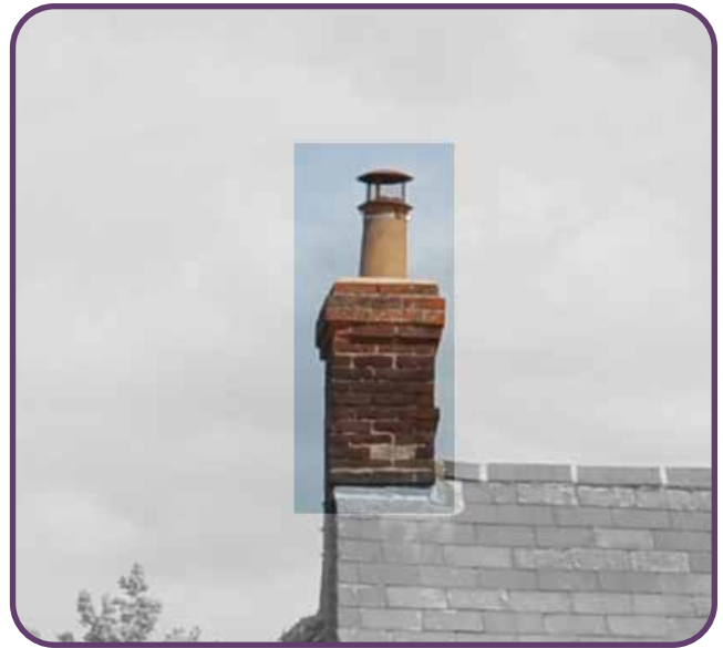
Figure 58: Chimney stack with red brick.
