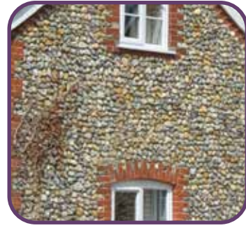
Flint stones with red bricks ornament
