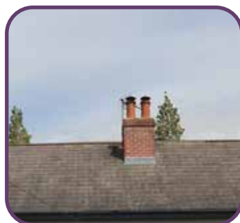
Chimney with red brick
