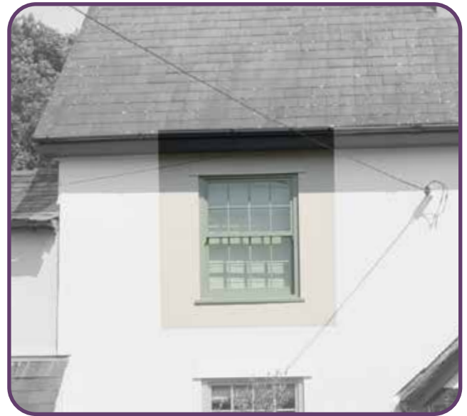
Figure 48: Multipanel sash window in Hargrave.
