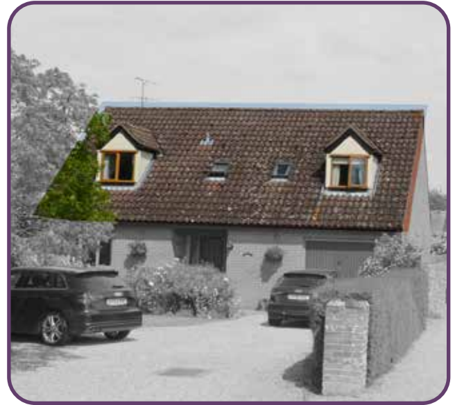
Figure 55: Pitched roof with pitched dormers.
