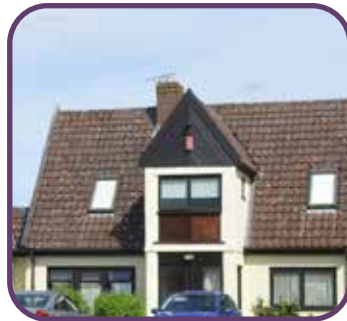
Pitched roof with pantiles
