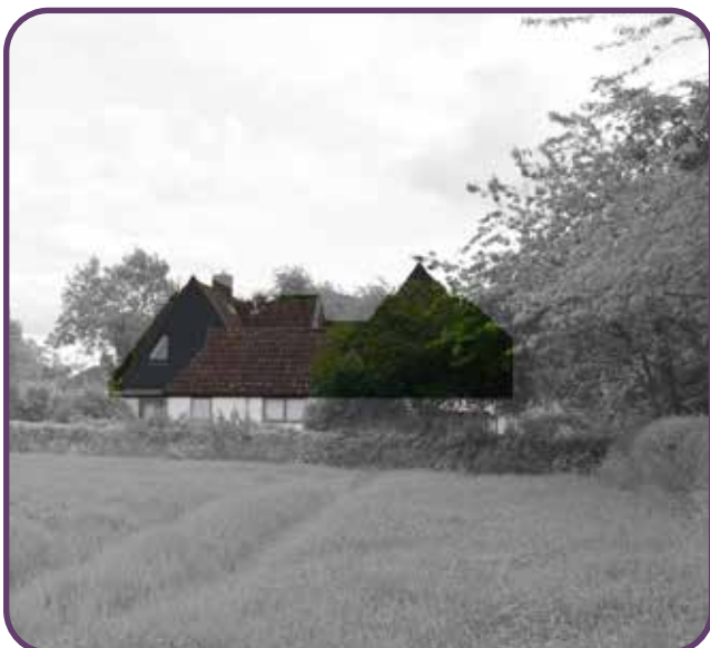
Figure 54: Articulated pitched and hipped roof.
