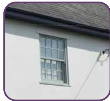
Sash window with timber frame
