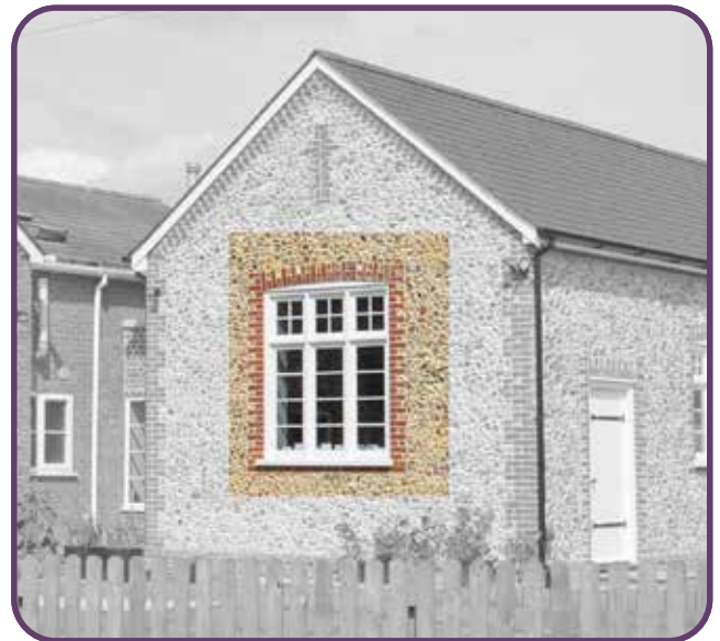
Figure 49: Casement window in Hargrave.
