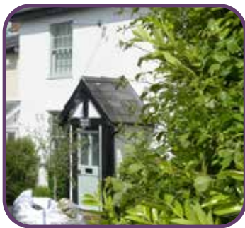
Typical porch door
