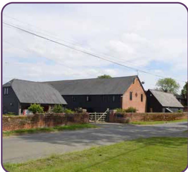
Figure 36: Grove Farm Barn on Wickhambrook Road.
