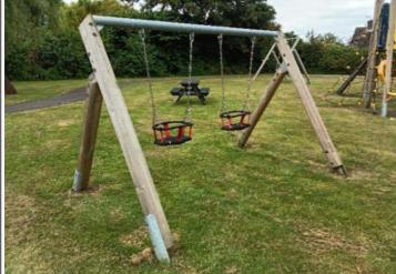
Finding: The swing seat frames are corroding
