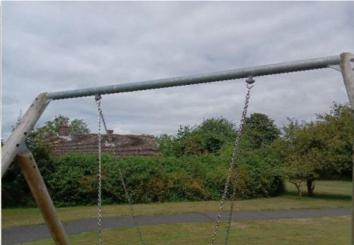
**Finding:** Swings of this design should have a secondary Action: Monitor use and check the joint and fixing security safety mechanism fitted to prevent collapse of the seat in the regularly event of a joint failure to comply with BS EN 1176 Part 2,
